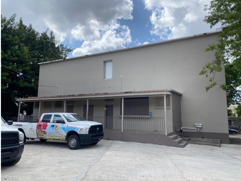
Description : BLDG1- Back side
