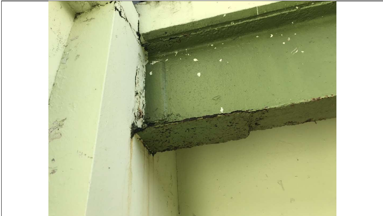
Picture 7 - Steel structure connections and sections with advanced corrosion conditions
