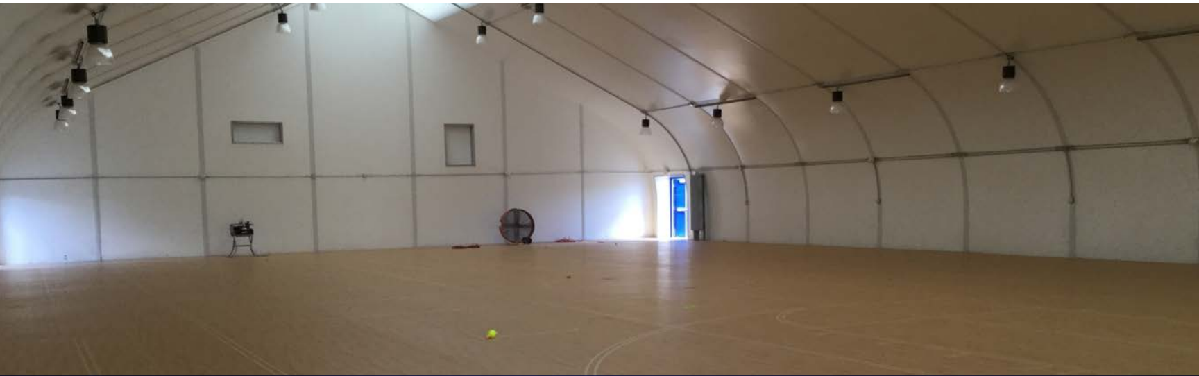
U.S. Virgin Islands Schools Program (FEMA funded program involving more than 240 new temporary classrooms and 19 new Sprung structures covering 16 school and other sites in two school districts on three islands)
