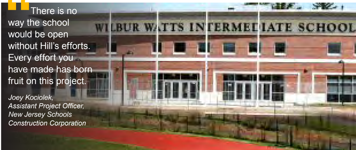
Hill supported the New Jersey Schools Construction Corporation on its $436M reconstruction and renovation program.
