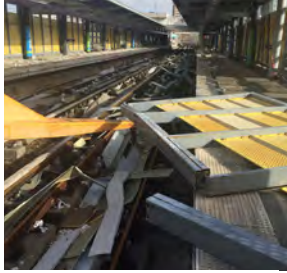
Tren Urbano PMO: $250M in federal funding
