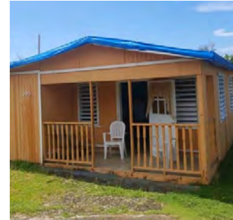
PR STEP: Completed 22,000+ single-family home repairs
